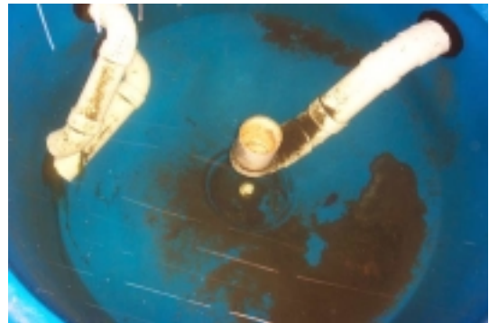
Top view of a DIY settlement chamber showing entering lines (left) and exit line (center) with settled solids
